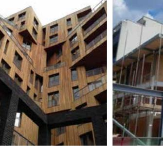
At ten storeys on completion this development was the tallest A single storey basement is provided with a secant piled wall, hybrid CLT building in Europe. The overall form steps and rotates which acted as the temporary water cut off to the adjacent up the building to create a complex and dynamic geometry. Wenlock Basin during construction.
