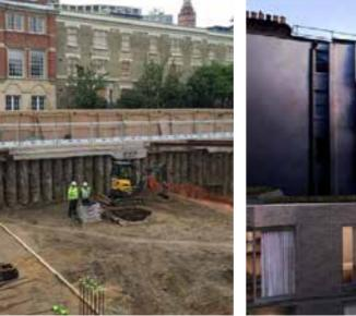
This boutique development consists of 28 apartments and three A concrete frame with a central stability core forms all but the townhouses in London's West End. top floor, which is constructed in lightweight steel frame to provide a large open plan penthouse.
