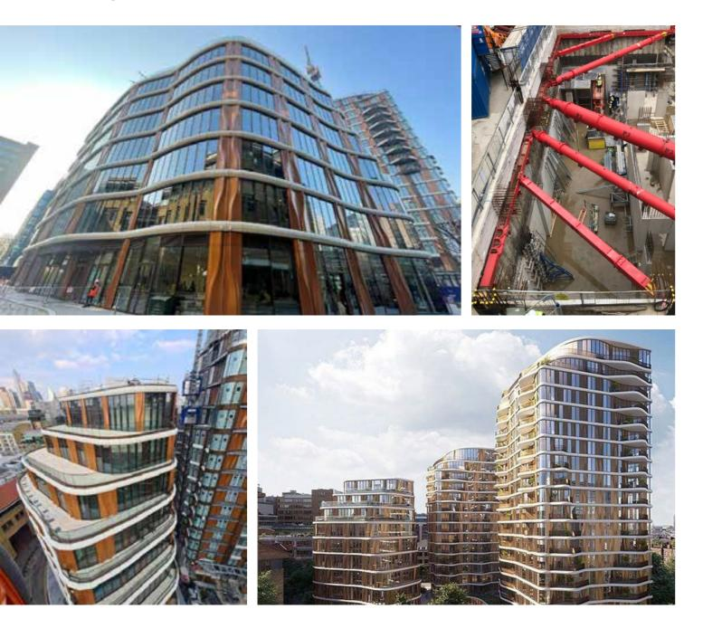
This substantial mixed-use development provides 163 residential units, office, retail and cultural facility space over three blocks with a double basement and landscaped podium. The two taller towers are residential, with in-situ flat slab construction using blade columns concealed within partitions. A transfer deck at ground floor allows a change in grid which maximises car parking spaces within the basement.
